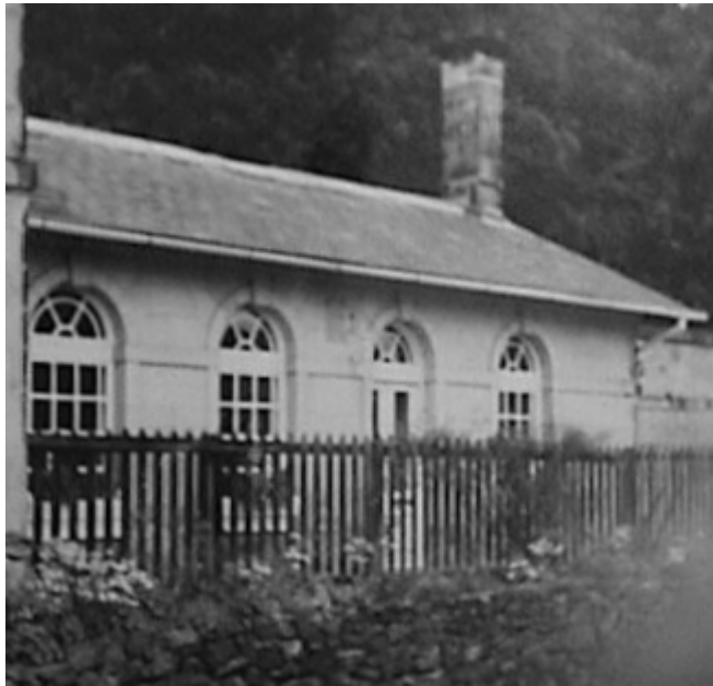
Detail of the railway face of the platform range.
