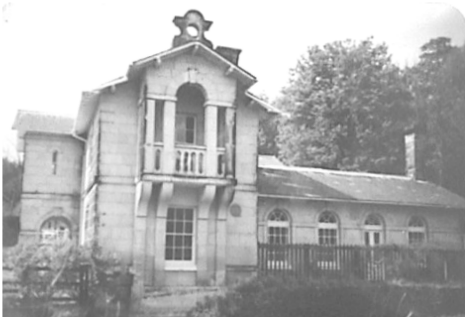
View of the railway faces of the main range and the platform range.
